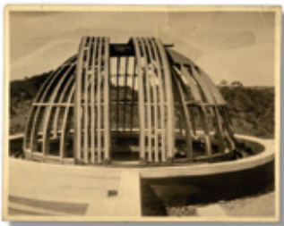
Mountain Boulevard Construction
